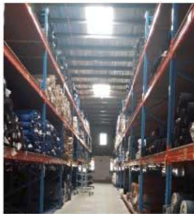
Skylights replace light bulbs in TAL's warehouse.
