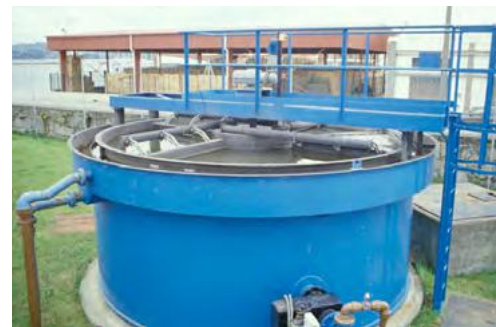
Elements of a DAF system with a circular flotation chamber Source: Advanced Energy Solutions SAE Ltda
