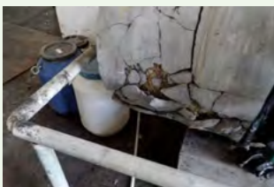
Damaged insulation
