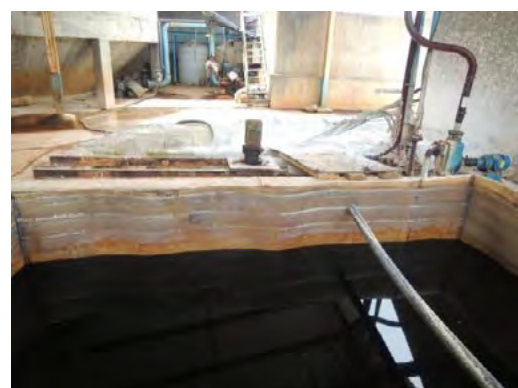
pH regulation system on a textile mil ETP (Zhejiang Lifeng 100 m 3 /h)
