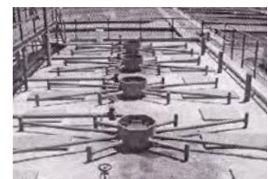
Influent distribution structures in: a circular reactor (left side) and a rectangular reactor (right side)
