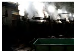
Steam leakage from a batch drying machine
