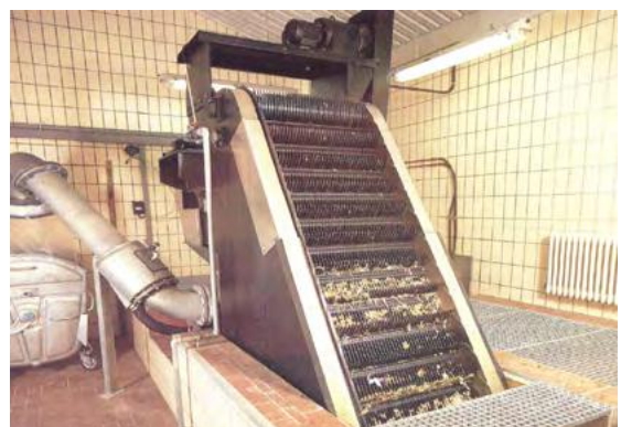
Self-cleaned step fine screen scheme
