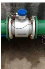
Installation of water flow meter in the waste water line of an audited mill
