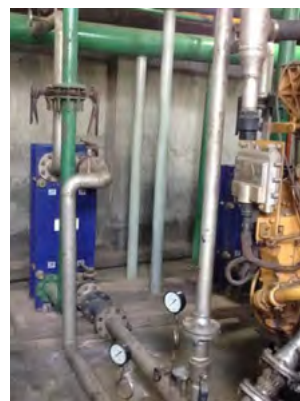
Water to water heat exchanger in a gen set of audited mill
