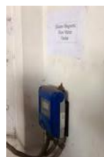
Installation of water flow meter in the waste water line of an audited mill
