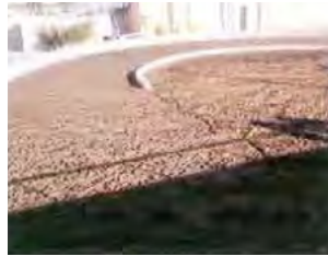
Biological reactor with foams after a period of stable performance Source: University of A Coruña
