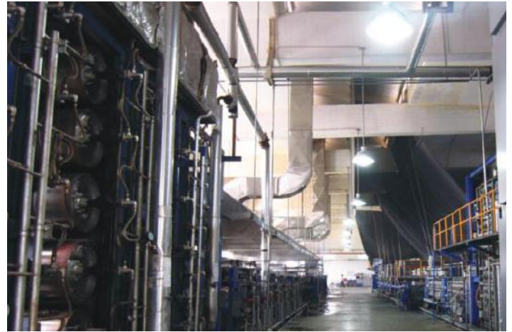
Better Insulation of steam pipes and valves
