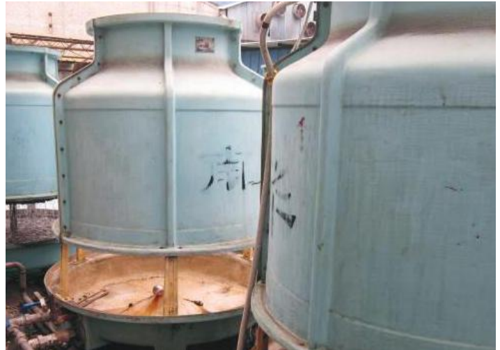
Inactive cooling water towers after reforming cooling system
