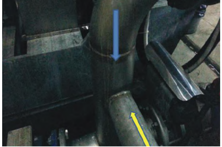
Collect rinsing water and reuse it for production after simple filtration and sediment
