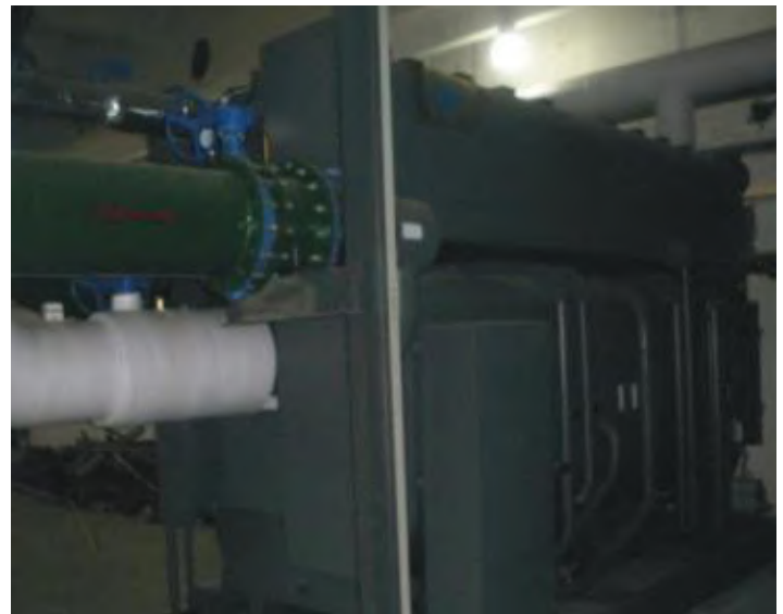
Lithium bromide air conditioner that uses condensate
