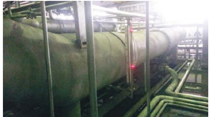
Insulation of dye vats
